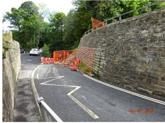
View look north along the street
