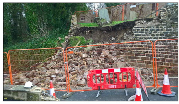
BOUNDARY WALL - CURRENT CONDITION
